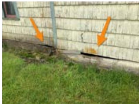
Skirting Wood Rot (Representative Picture)
