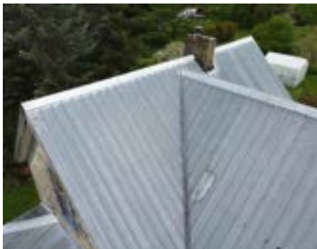
Right Side Roof - Side B
