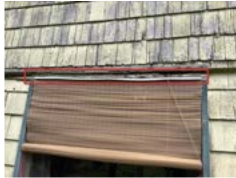
Siding/Trim Wood Rot (Representative Picture)
