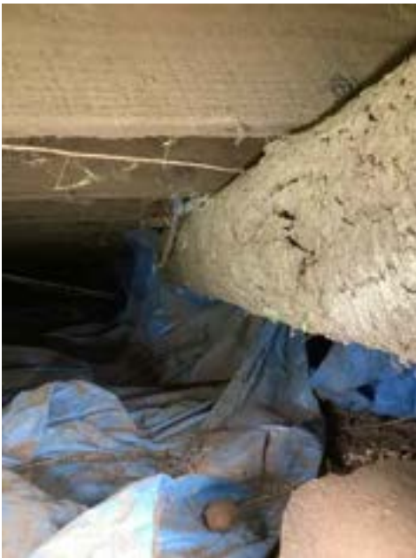
Limitations/Obstructions - Crawl Space (Representative Picture)
