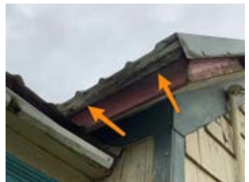
Multiple Roofing Layers (Representative Picture)
