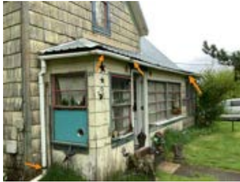
Gutter System Damaged/Not Present (Representative Picture)
