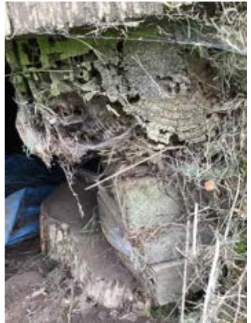
Limitations/Obstructions - Crawl Space (Representative Picture)
