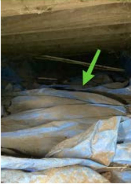
Vapor Barrier - Crawl Space (Representative Picture)
