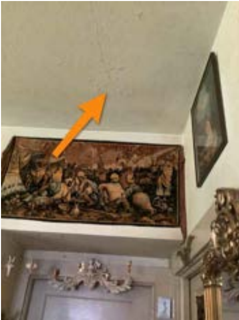
Smoke Detector(s) Not Present - First Floor (Representative Picture)
