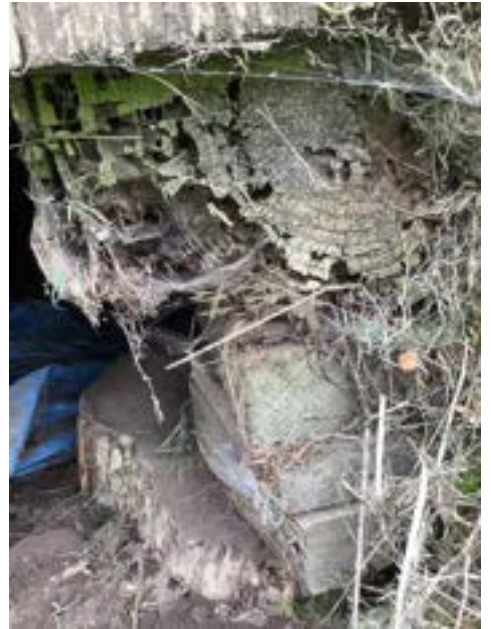
Limitations/Obstructions - Crawl Space (Representative Picture)
