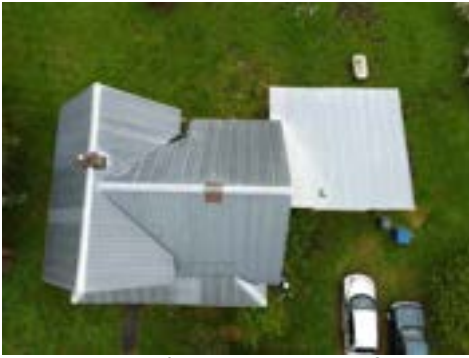
Limitations/Obstructions - Roof (Representative Picture)
