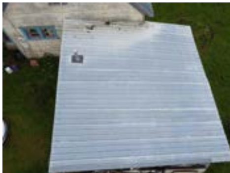
Flat Roof Structure - Side B
