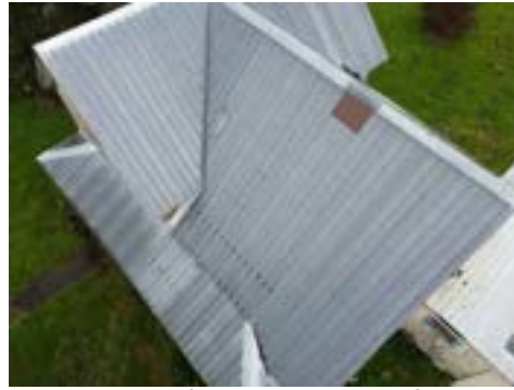
Limitations/Obstructions - Roof (Representative Picture)
