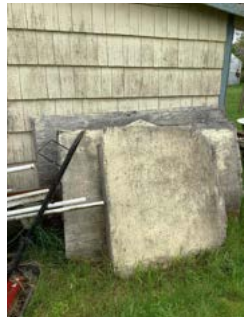
Wood in Contact With Siding - Side B
