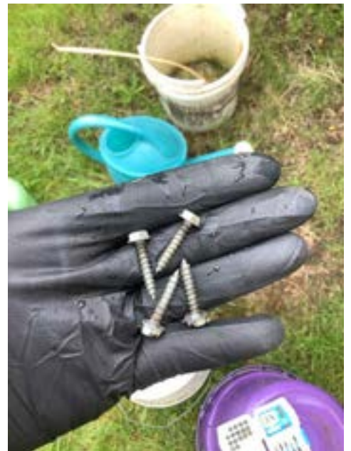
Incorrect Type of Panel Cover Fasteners - Side B
