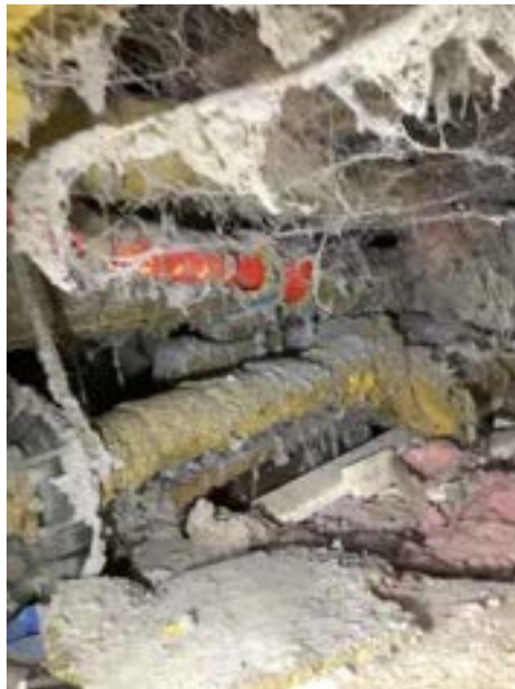
Limitations/Obstructions - Crawl Space (Representative Picture)
