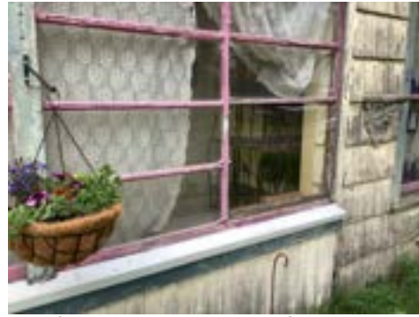
Window Trim/Frame Wood Rot (Representative Picture)
