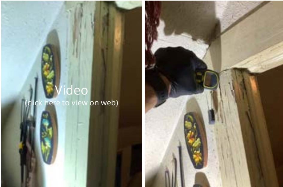
Signs of Moisture Damage - Bedroom (Second Floor)
