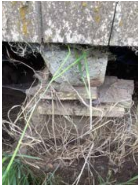
Limitations/Obstructions - Crawl Space (Representative Picture)
