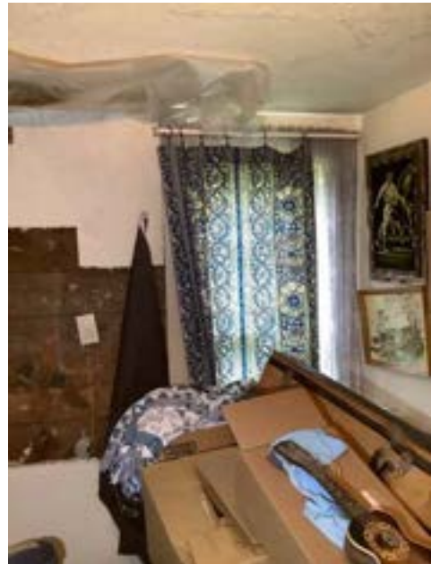
Limitations/Obstructions - Interior (Representative Picture)
