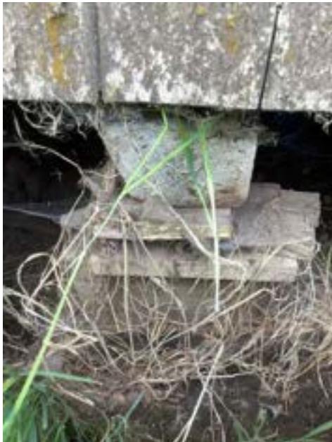
Limitations/Obstructions - Crawl Space (Representative Picture)
