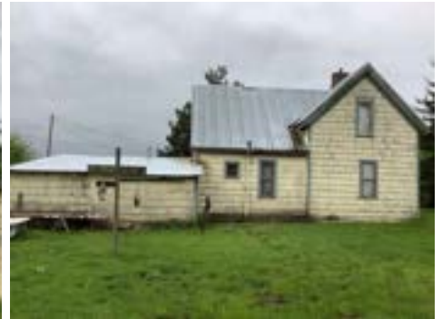
Back Side of the Home - Side C (North)
