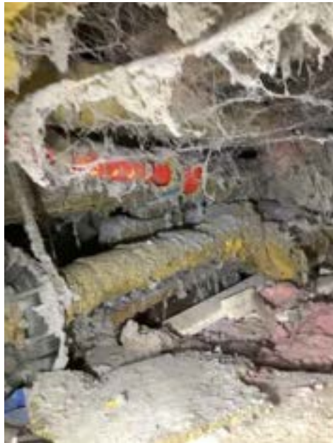
Limitations/Obstructions - Crawl Space (Representative Picture)
