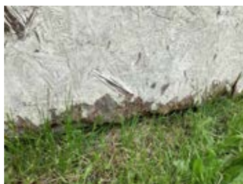
Garage Door Wood Rot - Side B (Representative Picture)
