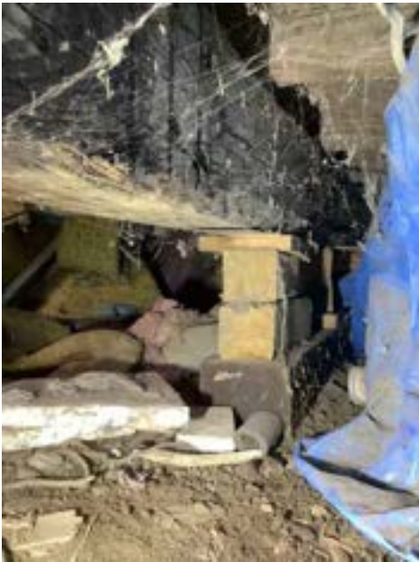
Limitations/Obstructions - Crawl Space (Representative Picture)
