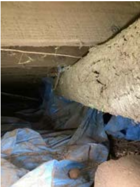
Limitations/Obstructions - Crawl Space (Representative Picture)
