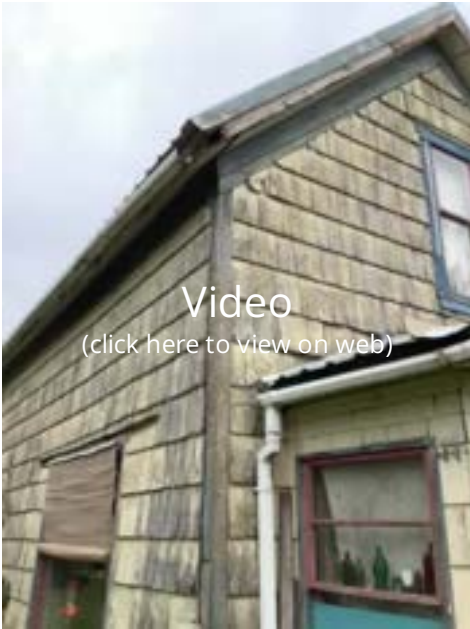
Gutter System Damaged/Not Present (Representative Picture)
