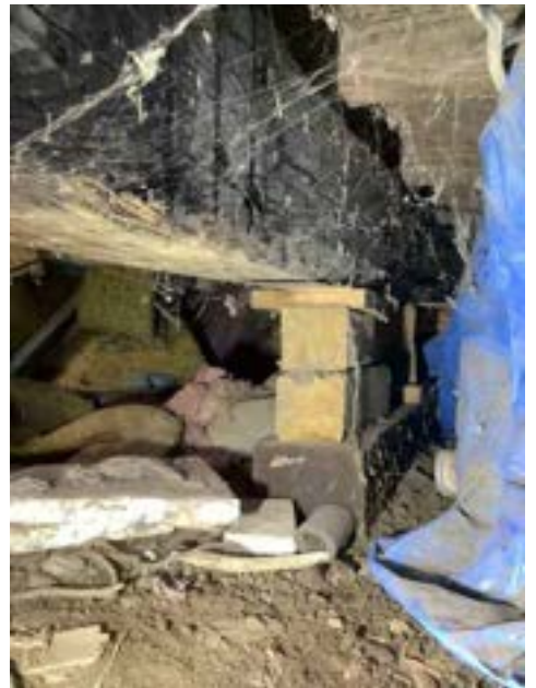
Limitations/Obstructions - Crawl Space (Representative Picture)
