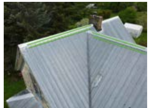
Ridge Vent(s) (Representative Picture)
