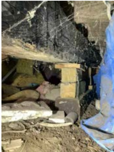
Limitations/Obstructions - Crawl Space (Representative Picture)
