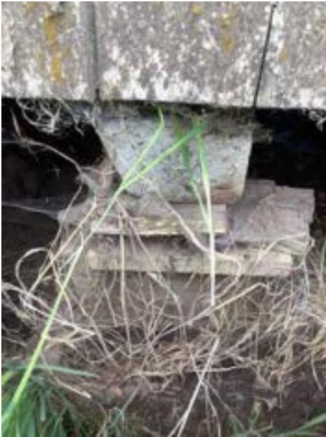
Limitations/Obstructions - Crawl Space (Representative Picture)
