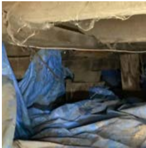
Limitations/Obstructions - Crawl Space (Representative Picture)
