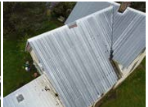
Back Side Roof - Side C
