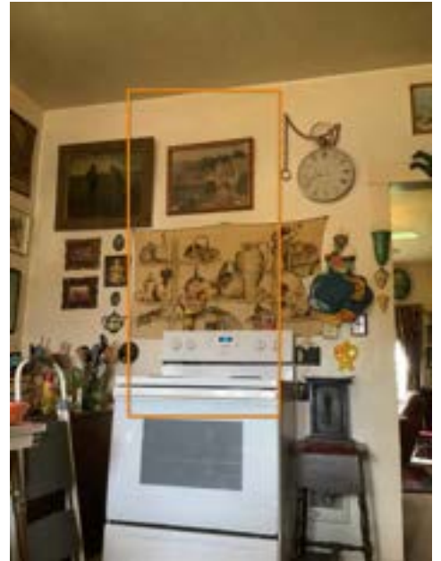
Range/Oven Exhaust System Not Present - Kitchen (First Floor)
