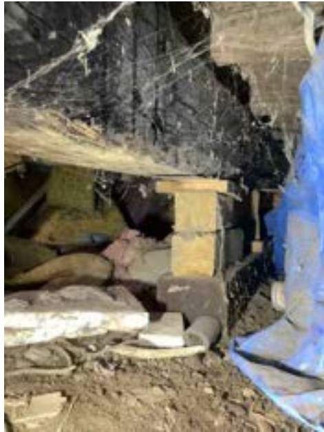
Limitations/Obstructions - Crawl Space (Representative Picture)
