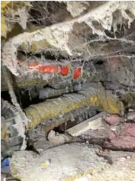
Limitations/Obstructions - Crawl Space (Representative Picture)
