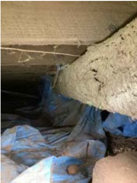
Limitations/Obstructions - Crawl Space (Representative Picture)
